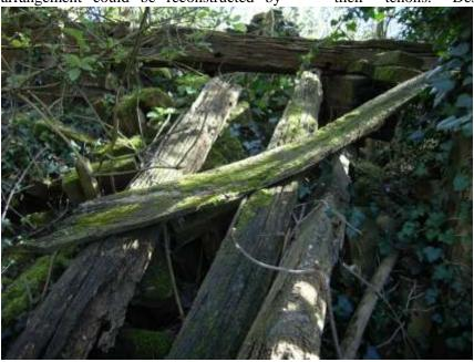
Illus. 3 An external wall brace in the western elevation, still trenched across the studs despite its precarious angle.
