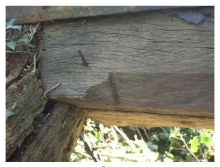
Illus. 6 Detail of distinctive late-16<sup>th</sup> century chamfer stop to binding joists
