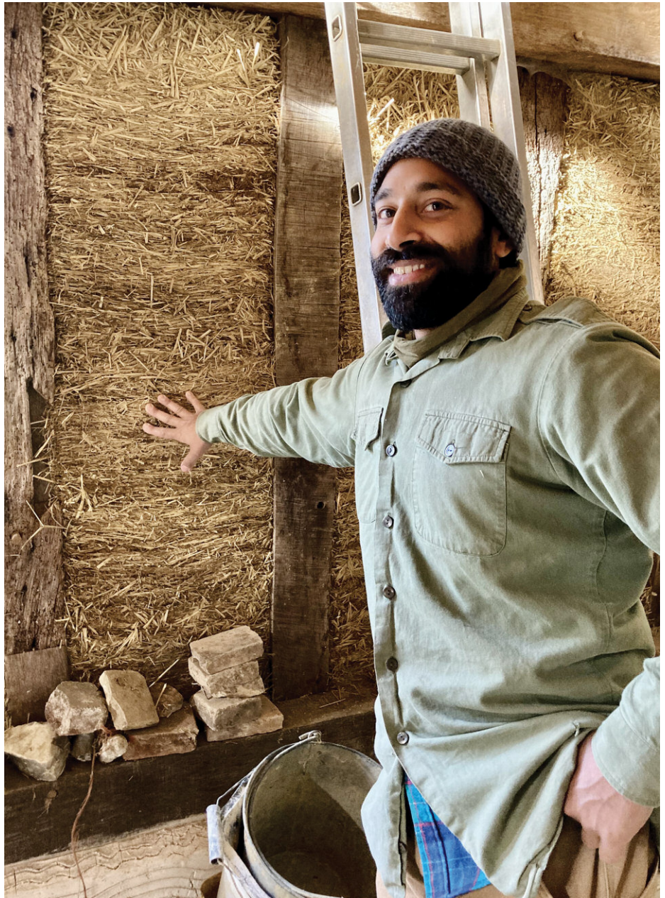
Going to the wall: Hiran Tailor showcases the light straw-clay insulation
