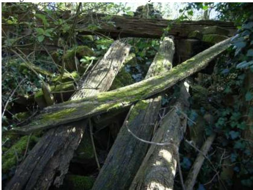
**Illus. 3 An external wall brace in the western elevation, still trenched across the studs despite its precarious angle.**
