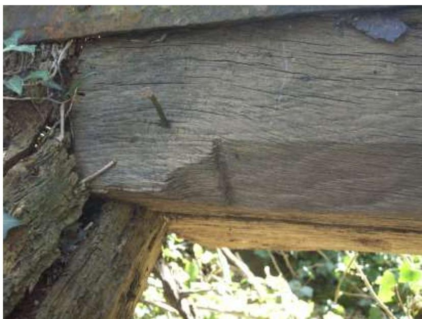
**Illus. 6 Detail of distinctive late-16<sup>th</sup> century chamfer stop to binding joists**
