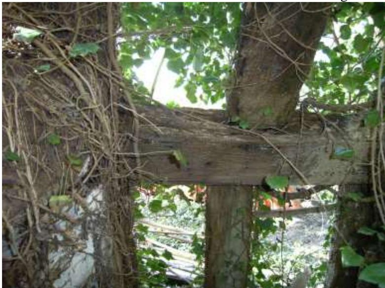
**Illus. 4 The south-western corner of the later hall, showing intact mid-rail and studs with secondary cross-passage screen to left.**
